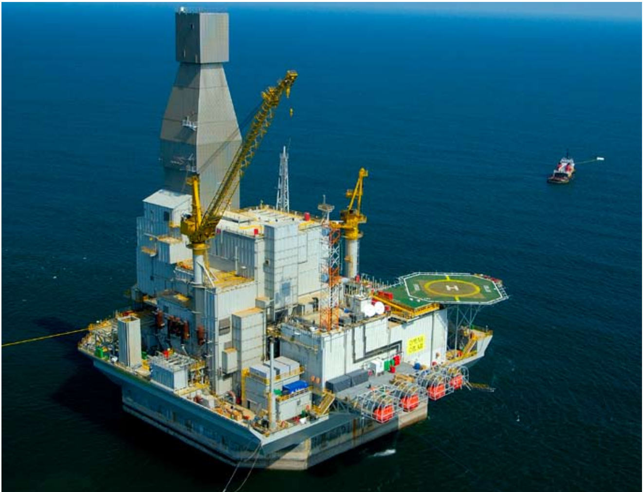
Orlan offshore platform, Sakhalin-1
