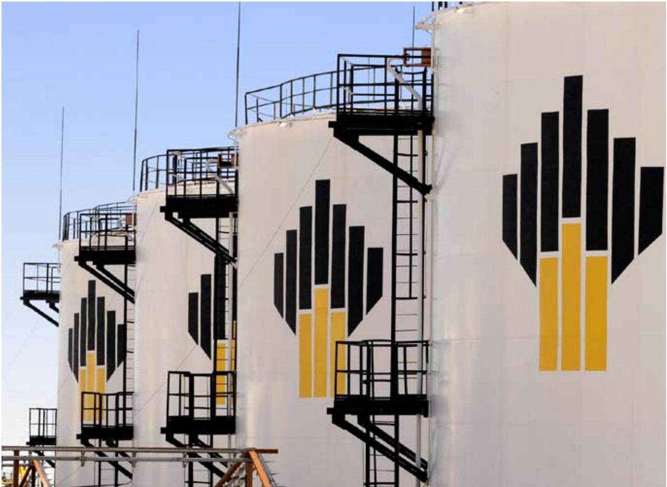
Purneftegaz fuel and lubricants base – tank farm
